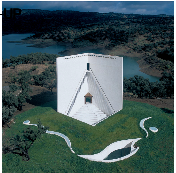
Built beneath the ground, sinuous walls and a smooth open interior are lit from skylights while the earth provides insulation from both heat and cold. A waterfall cascades into the home, which is further punctuated by patios. Photography by Michele Alassio. Image © Emilio Ambasz & Associates.
